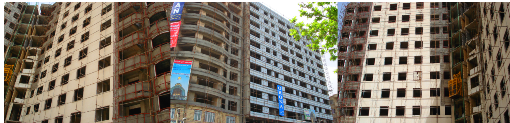
Fig. 6 A residential tower with 80 houses
